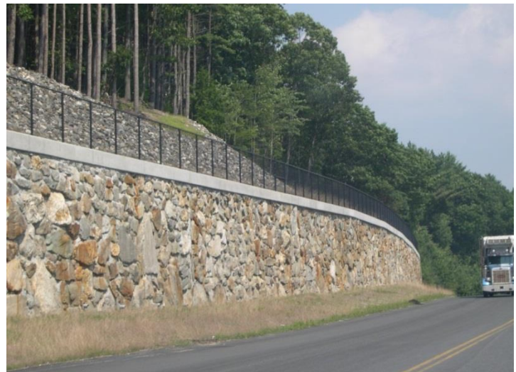
Relocated portion of Route 2 in Erving that was completed as part of the Route 2 East Safety Improvements.
