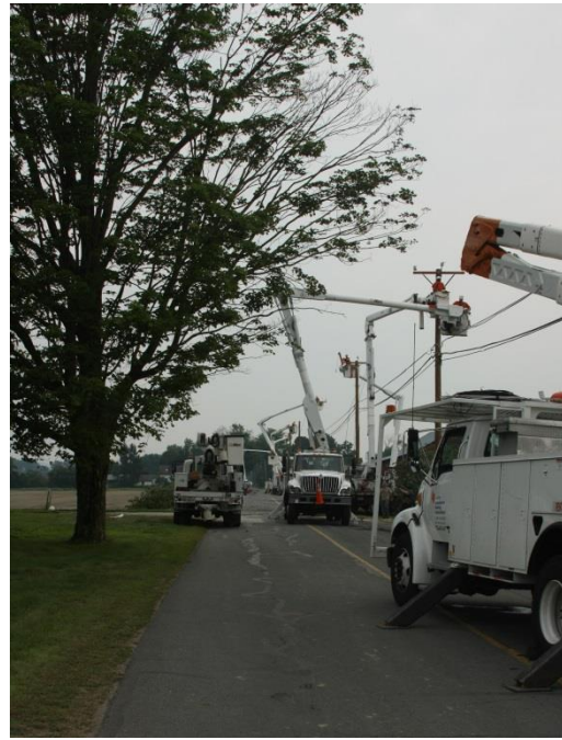
Utility trucks repairing power lines after a damaging storm in Whately.
