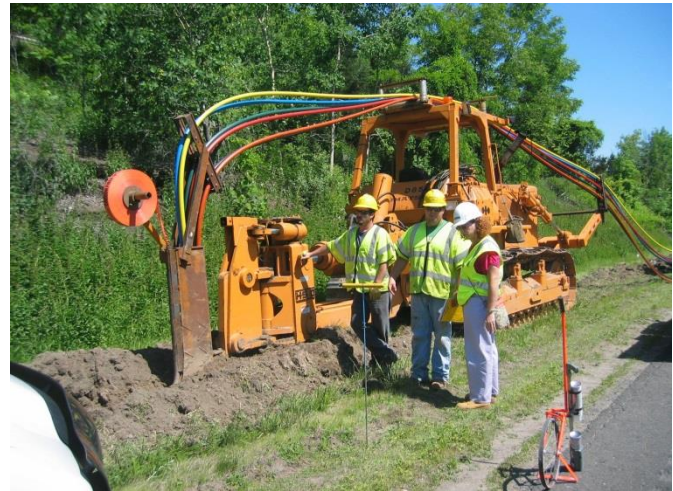
Installing broadband conduit along I-91.
