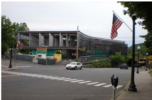
Regional Transit Center under Construction
