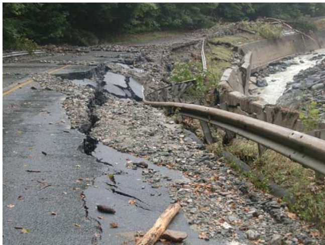
Flooding and Road Damage from Hurricane Irene, 2011
