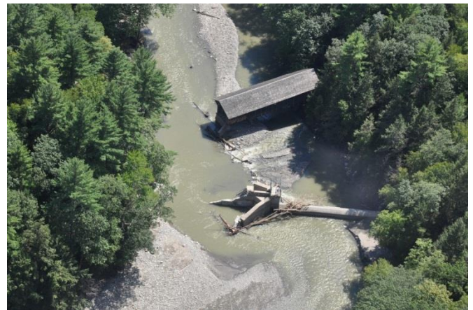
Cultural resources can be vulnerable to flooding, as was seen during Tropical Storm Irene, which knocked the Eunice Williams Covered Bridge in Greenfield from its footings.
