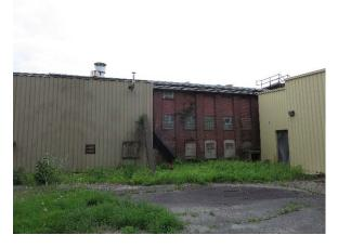
likely due to Building 3's proximity to the wall and shielding it from significant sunlight, therefore not allowing moisture to evaporate in a timely manner.
