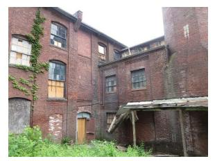
The brick masonry building is currently in fair condition, however with the water ingress into it from the roof collapse, deterioration will likely accelerate. The brick chimney appeared to be in fair to poor condition. Approximately one third to one half of the chimney has been previously reinforced and there are signs of deterioration throughout its height.
