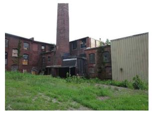
The exterior of the building is not exposed very much as it is surrounded by other buildings on three sides. The north edge of the building is exposed to view and is in poor condition. Water damage is apparent and vegetation growth has started. The mortar is extremely soft and has failed in several locations where brick units have fallen out of the wall.
