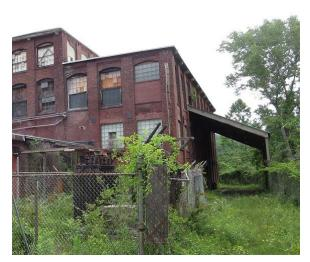
are several exposed pipes along the wall and Building 5c provides an enclosed delivery area; the brick along this wall is also in fair to poor condition.
