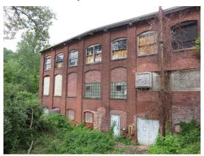
The exterior brick walls are generally in poor condition. There are several locations throughout the building's perimeter where loose or soft mortar was found and numerous areas where brick units are loose or have been lost.
