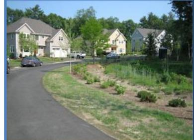
Example of a subdivision that has incorporated LID elements, including a narrow roadway and a bioretention area.
