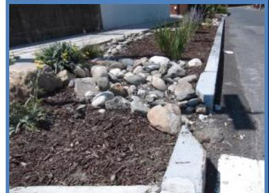
Retrofit of an existing street to include bioretention areas between the roadway and sidewalk.
