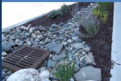
Left: A bioretention area in the tree belt on Olive Street complements the traditional storm drain.
