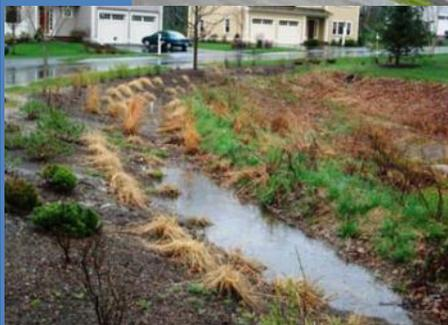
Left: Stormwater being treated in a road-side bio-retention area.
