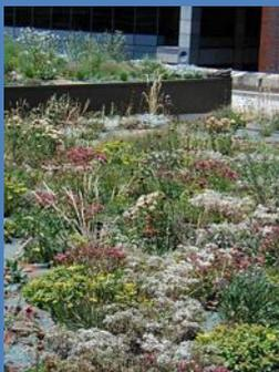
Vegetative layer grown on a roof reduces and slows stormwater runoff and filters pollutants.
