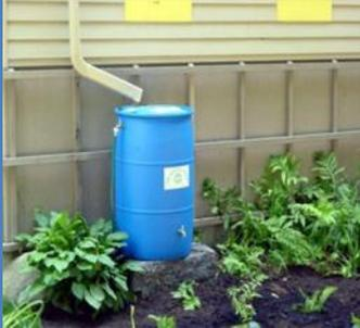
Runoff from roofs is collected in rain barrels or cisterns for outdoor watering or for indoor non-potable uses such as toilet flushing.
