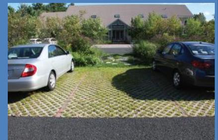
Photo: Chris Curtis. Porous pavers and asphalt at New England Environmental, Inc. Amherst, MA.
