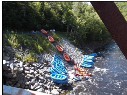
Stairway and boat slide, and platform used to access the Deerfield River.
