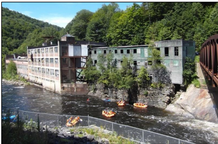
Rafters wait below the wood structure for all boats to be launched before going down the Deerfield River.
