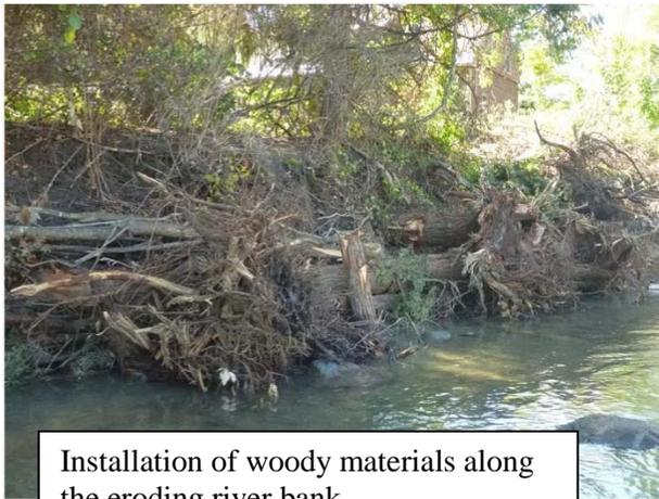
Installation of woody materials along the eroding river bank.
