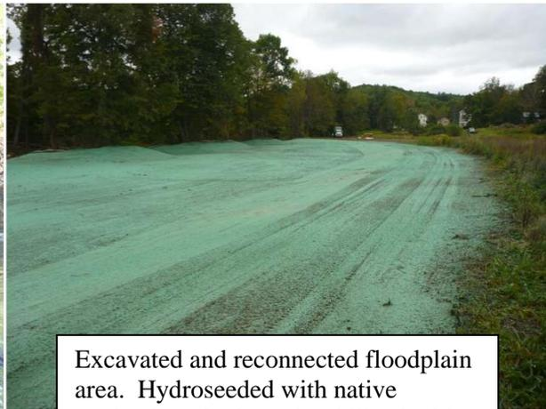
Excavated and reconnected floodplain area. Hydroseeded with native wetland seed mix and stabilized with jute netting.
