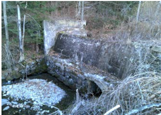
Although the dam on Foundry Brook is partially breached, it still acts as a fish barrier and hydraulic/flood barrier.
