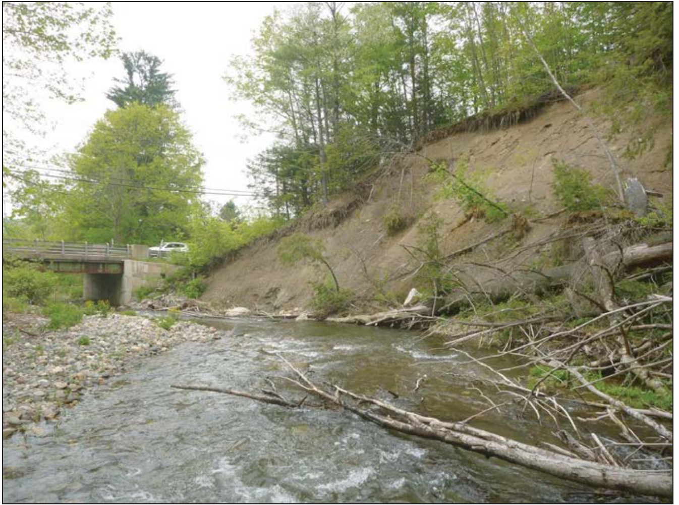
Lower Clesson Brook - photo of mass failure just upstream of Route 112 crossing on lower Clesson Brook.
