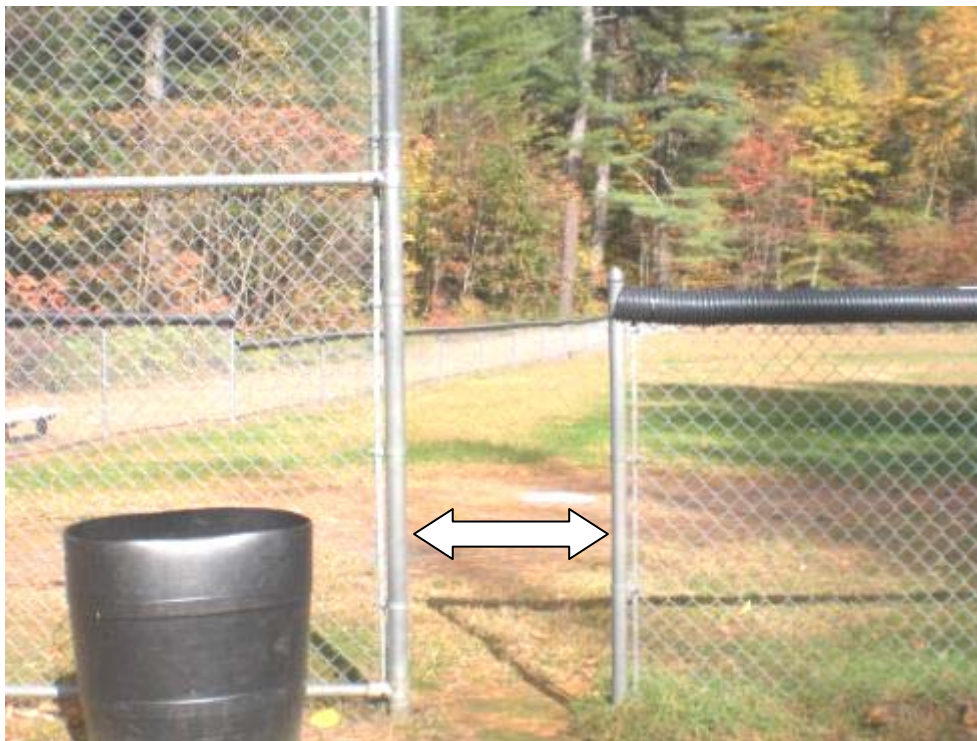
Less than 36" ADA allowable fence openings to the ball field at Buckland Recreation Area prohibits access via wheelchair.
