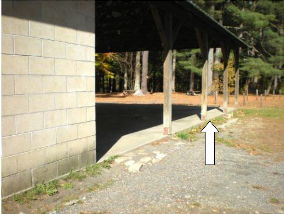
Greater than 6" allowable edges on the Buckland Recreation Area pavilion slab prohibits access via wheel chair.
