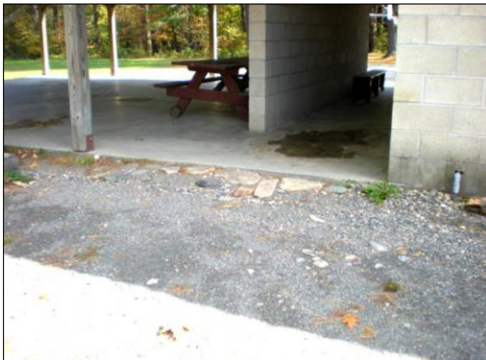
Uneven ground on the path to Buckland Recreation Area pavilion makes access via wheel chair challenging.
