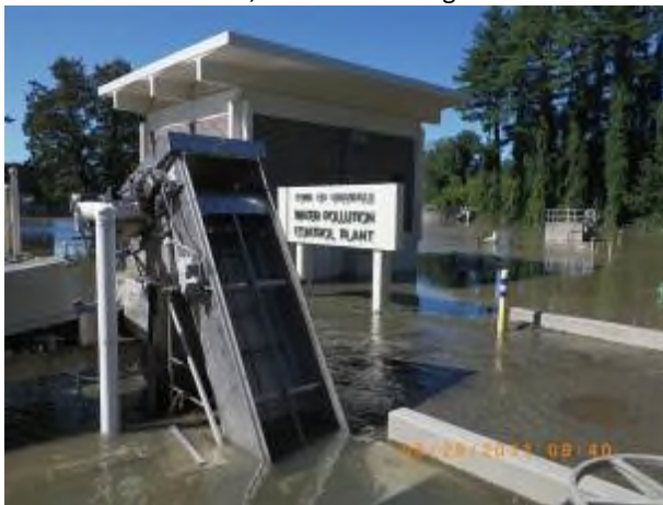
The Wastewater Treatment Plant was flood-proofed to elevation 140 feet but Irene's flooding topped elevation 142 ½ feet.
