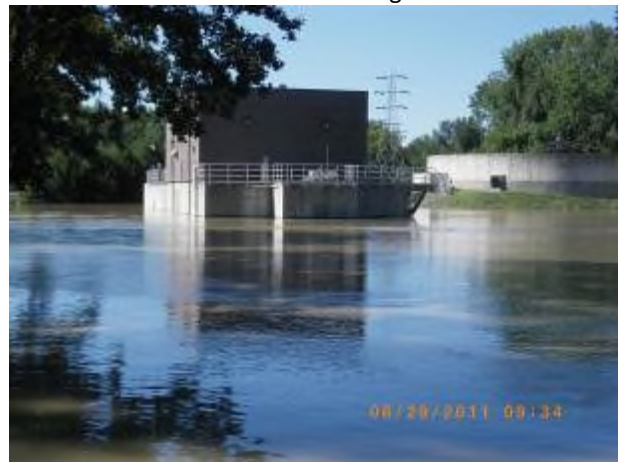
The Wastewater Treatment Plant was flood-proofed to elevation 140 feet but Irene's flooding topped elevation 142 ½ feet.
