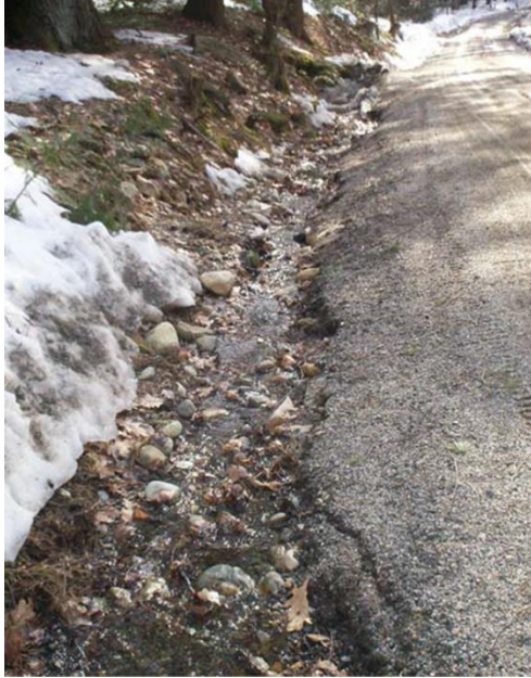
Above left: one of the sites on Four Mile Brook Road prior to the project. Above right: The same location after installation of a rock-lined swale that collects, slows, and filters stormwater runoff from the road, helping to keep the roadway edge intact.
