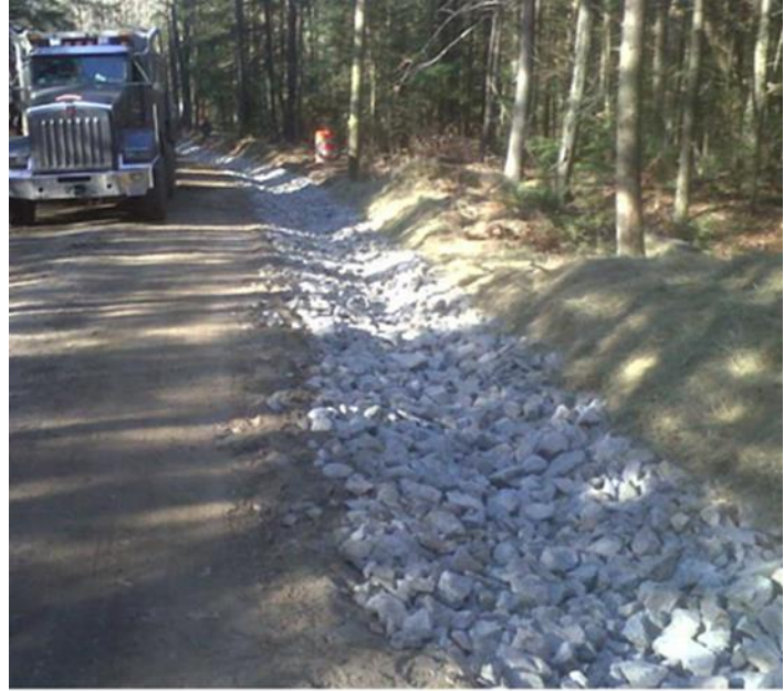
Above left: one of the sites on Four Mile Brook Road prior to the project. Above right: The same location after installation of a rock-lined swale that collects, slows, and filters stormwater runoff from the road, helping to keep the roadway edge intact.
