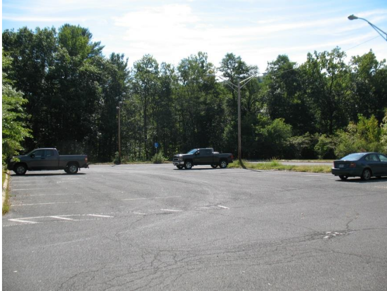
Figure 1. Charlemont Park & Ride Facility
