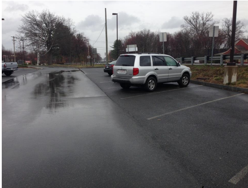
Left: The Whately Park and Ride lot on a rainy day. The porous asphalt in the parking stalls allows stormwater to infiltrate through. In contrast, rain is ponding in the drive aisle where non-porous asphalt was used.
