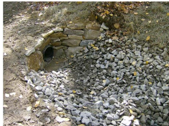
Above: Uncontrolled runoff scours and erodes an unpaved road. Below: A stabilized culvert inlet and rock drainage channel help slow and convey stormwater runoff away from the roadway.
