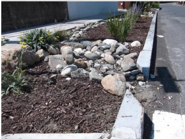
Top left: Olive Street before the tree belt was installed. Top right: Olive Street after the tree belt installation. The top photos are taken from the entrance to the JWO Transit Center. Bottom left: a curb cut allows stormwater from the roadway to enter the rock-lined swale which also traps sediment.
