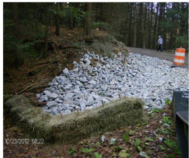
Above left: A natural stone headwall at the inlet end of a road culvert on Four Mile Brook Road. Above right: A ditch turnout on Four Mile Brook Road. These BMPs slow, filter and convey stormwater runoff from the roadway, reducing erosion and removing sediment before it enters the brook.
