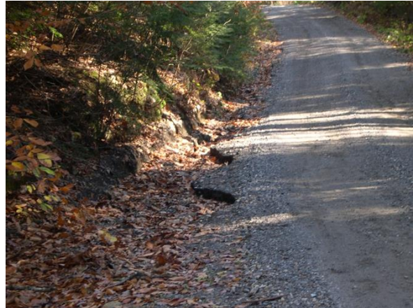
Above: Uncontrolled runoff scours and erodes an unpaved road. Below: A stabilized culvert inlet and rock drainage channel help slow and convey stormwater runoff away from the roadway.
