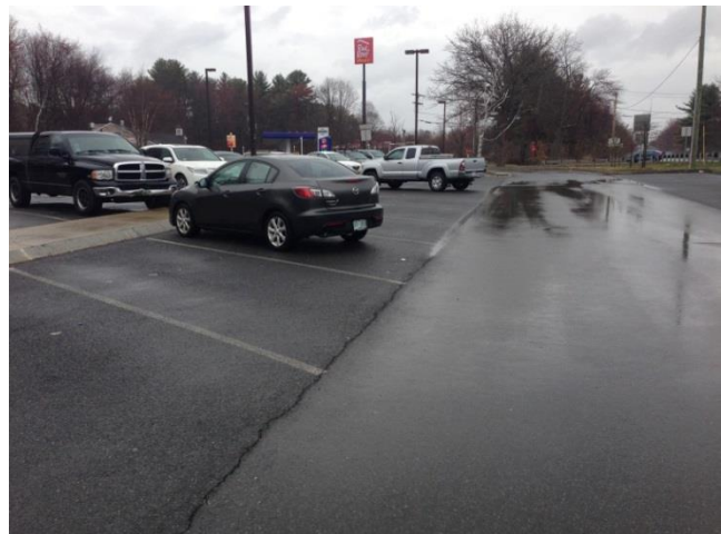
Porous asphalt is used for the parking stalls at the Whately Park and Ride Lot. The travel lane is constructed of traditional asphalt. Note the lack of ponding in the parking stalls during a rain storm.
