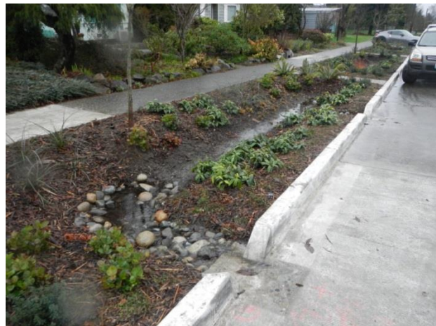
A stone pre-settling zone at the inlet to a bioretention swale allows sediment to settle out before runoff enters the swale. Image source: NACTO Urban Street Stormwater Guide
