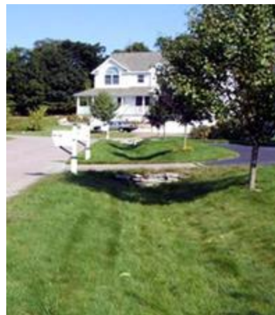
A roadside swale on a residential street collects and infiltrates stormwater runoff from the roadway. Source: MA Smart Growth / Smart Energy Toolkit
