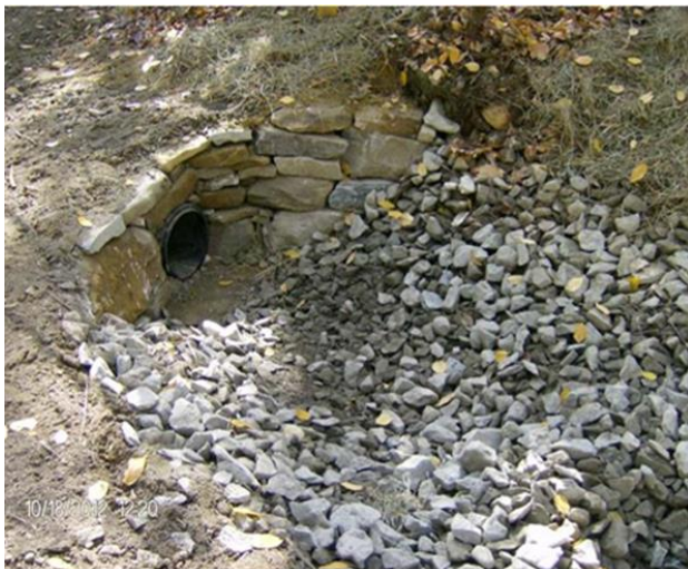
Above left: A natural stone headwall at the inlet end of a road culvert on Four Mile Brook Road. Above right: A ditch turnout on Four Mile Brook Road. These BMPs slow, filter and convey stormwater runoff from the roadway, reducing erosion and removing sediment before it enters the brook.
