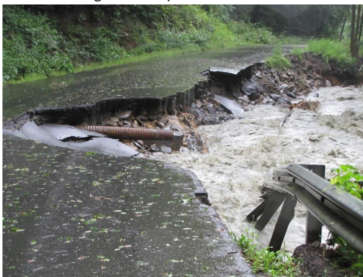
In 2011, flooding from Tropical Storm Irene caused massive damage to roads and infrastructure in western Franklin County, such as this road in Colrain.
