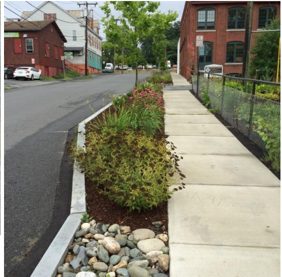
Top left: Olive Street before the tree belt was installed. Top right: Olive Street after the tree belt installation. The top photos are taken from the entrance to the JWO Transit Center. Bottom left: a curb cut allows stormwater from the roadway to enter the rock-lined swale which also traps sediment.
