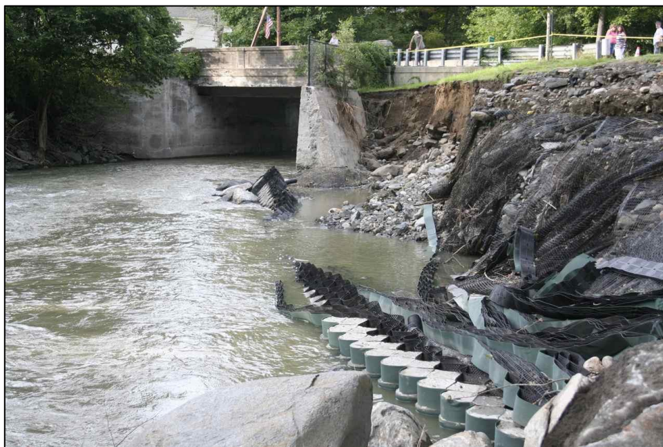
Damaged gabion retaining wall below the Route 116 Bridge along the South River, after Tropical Storm Irene in 2011
