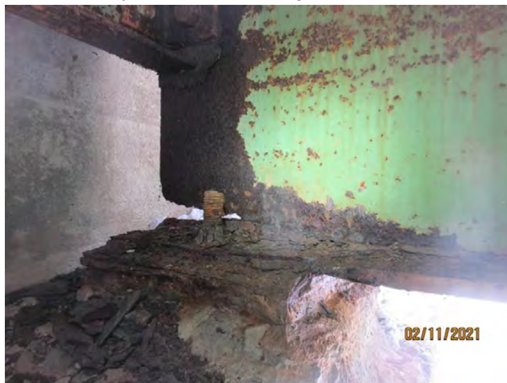
2021 Photo of Beam 5 North End:
