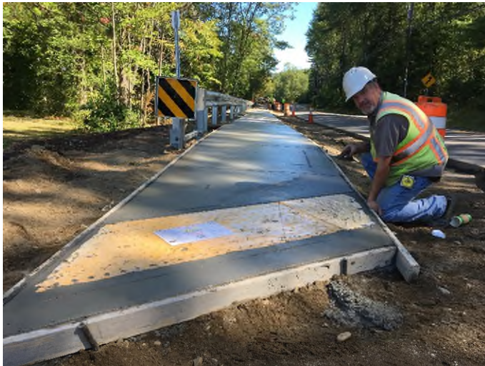
Sidewalk under construction in Erving.
