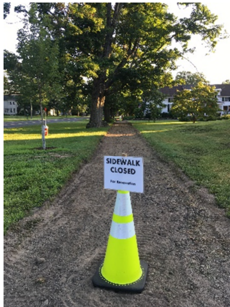
South Main Street sidewalk under construction in Sunderland.
