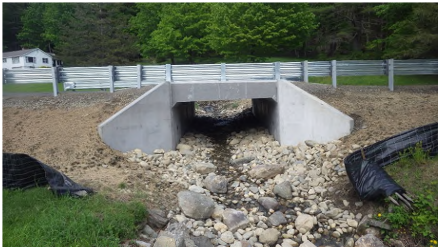
Before and After Pictures of a Culvert Replaced in Colrain to Accommodate Increased Rainfall Amounts
