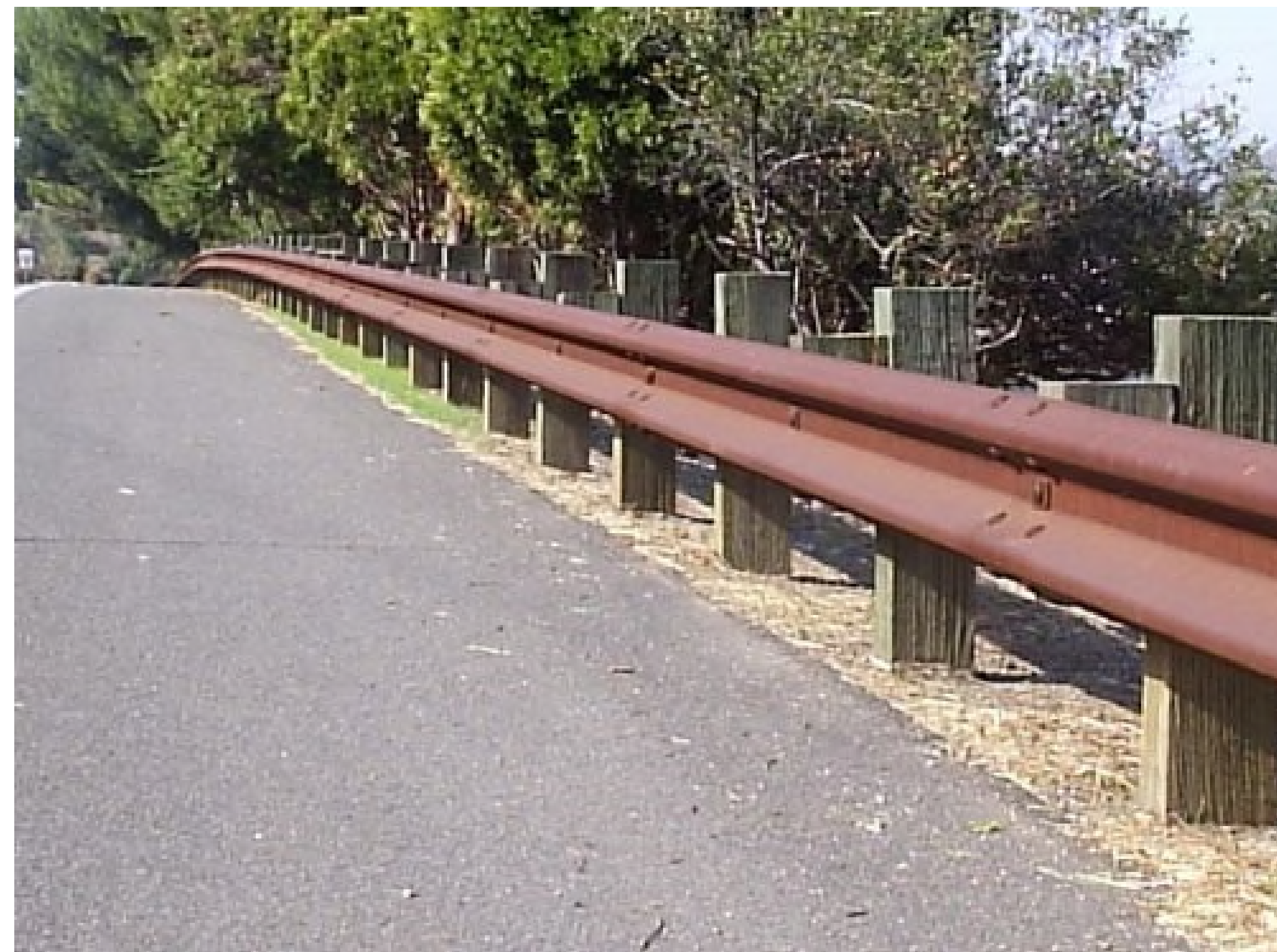
Weathered Steel W-Beam
